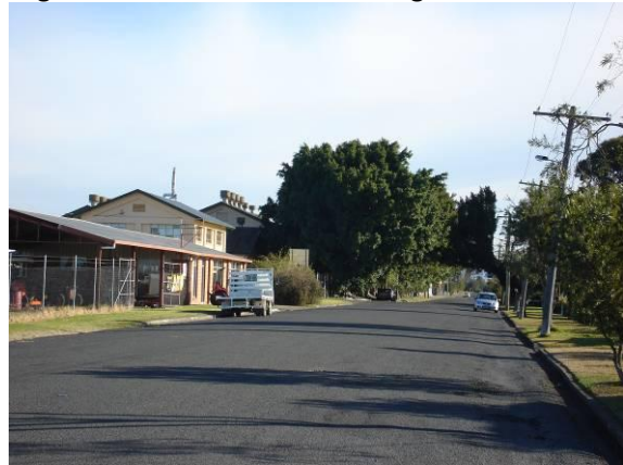
Figure 4.5 – Pitt Street looking west
